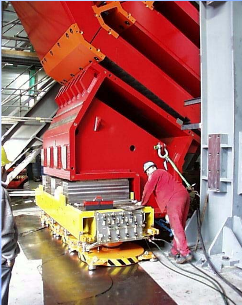
Magnet Support under installation
